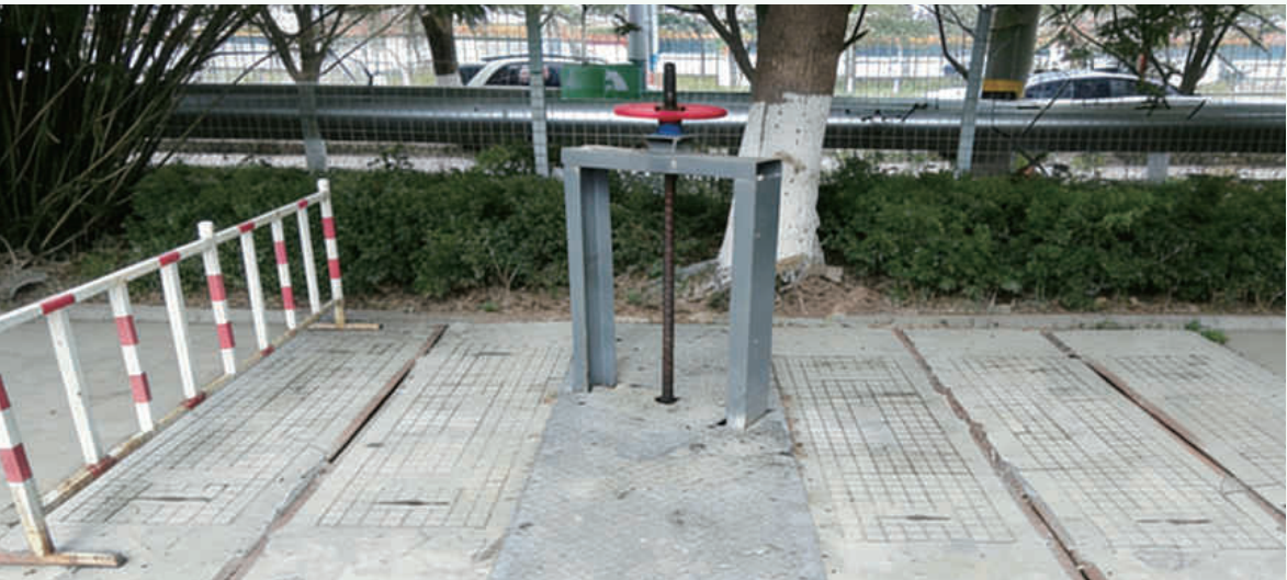
Rainwater Collection Basin on Site
